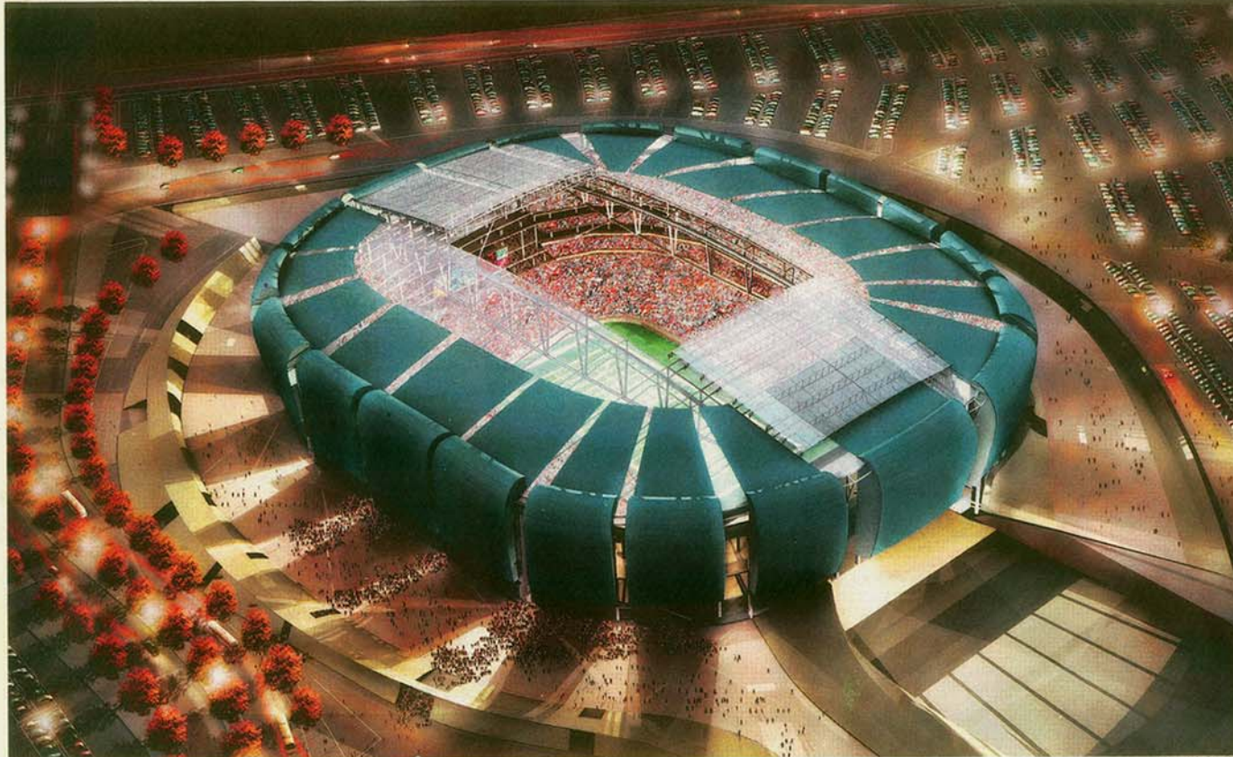
Peter Eisenman's stadium design for the Arizona Cardinals of the National Football League has a facade of shimmering aluminum panels and a field that can slide in and out of the arena as needed.
